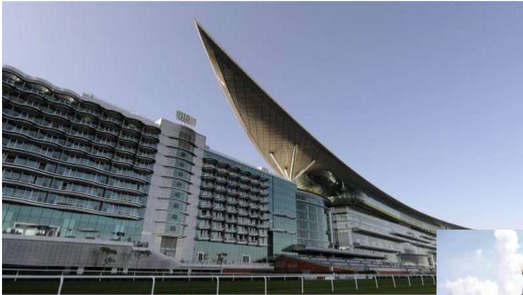
Meydan Hotel - Dubai Underground Cable Tunnel
