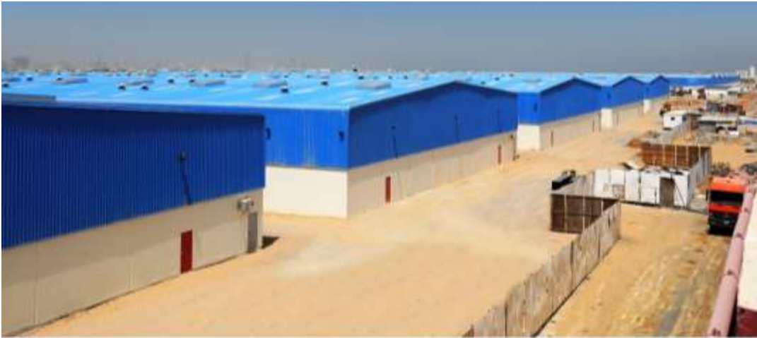
Ajman Free Zone Creek Development - 800 Warehouses
