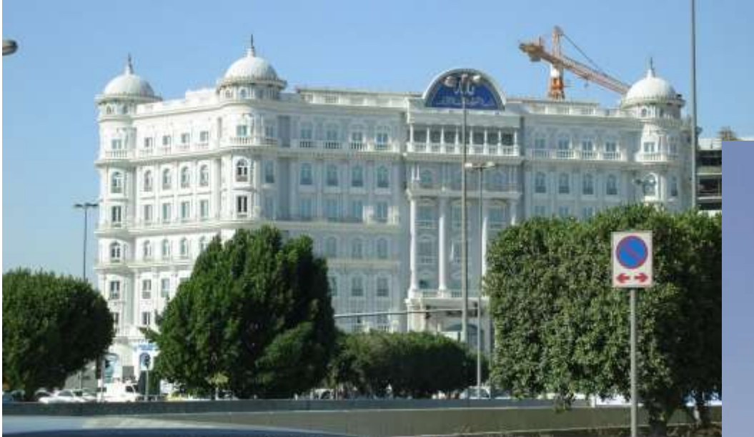
Al Serkal Building, Airport Road, Dubai 2B+G+8 - Commercial Bldg
